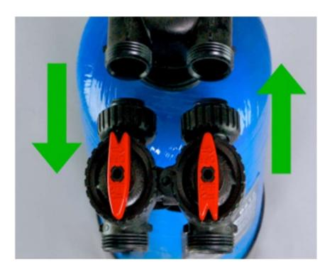
If the arrows are turned the wrong way, simply pull the arrow straight up off the peg, turn 180 degrees, and reattach by pushing the arrow back onto the peg. Reposition the second arrow in the same manner, if necessary.
