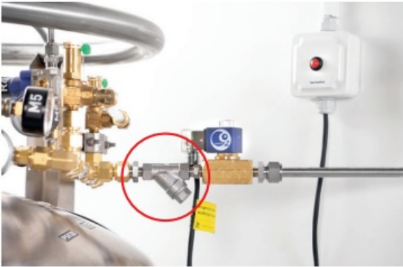
SMB and safety valve installed with filter
