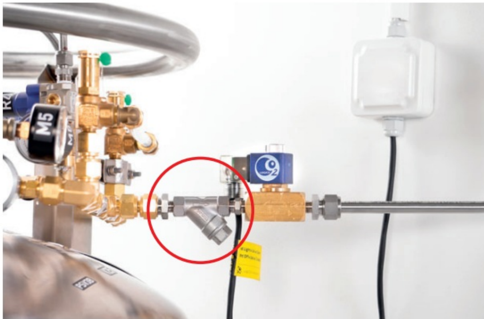
Enrichment Valve installed with filter
