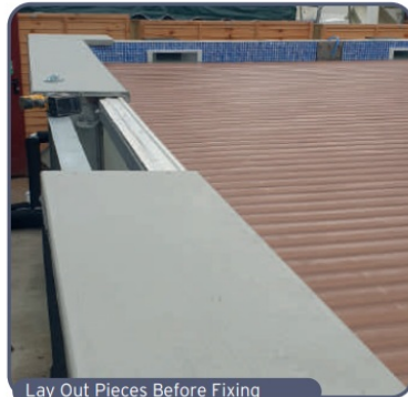
Lay Out Pieces Before Fixing
