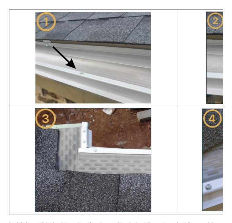
**Straight Runs:** Work left to right as viewed from the ground. Lay Leaf4go Micromesh completely flat over existing gutters with the front edge of the panel lined up with the top front edge of the gutter and the back edge lying on the drip edge.
