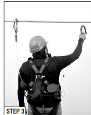
STEP 3 For lateral movement connect the second leg of the lanyard successive anchorage point.
