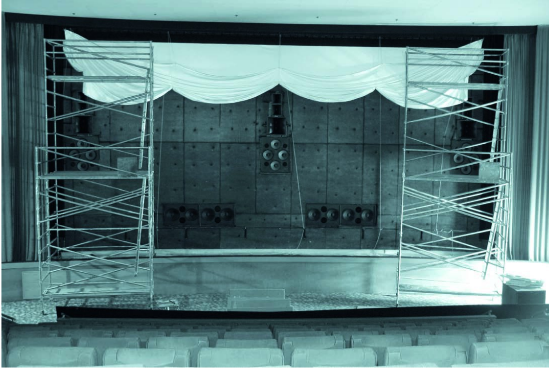
Wallis Cinema, Noarlunga, South Australia. Commercial cinema installation featuring a 'Baffle Wall', Krix Commercial 4-Way loudspeakers, and dual 18" subwoofers.
