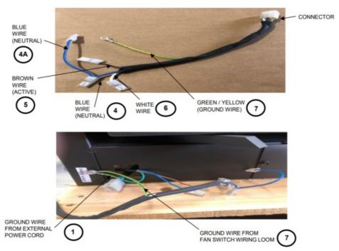
3. USE THE SELF TAPPING SCREW AS ATTACHED AND LABELLED FOR GROUND WIRES, SCREW BOTH GROUND WIRES FROM THE EXTERNAL POWER CORD AND FAN SWITCH WIRING LOOM AS SUPPLIED.
