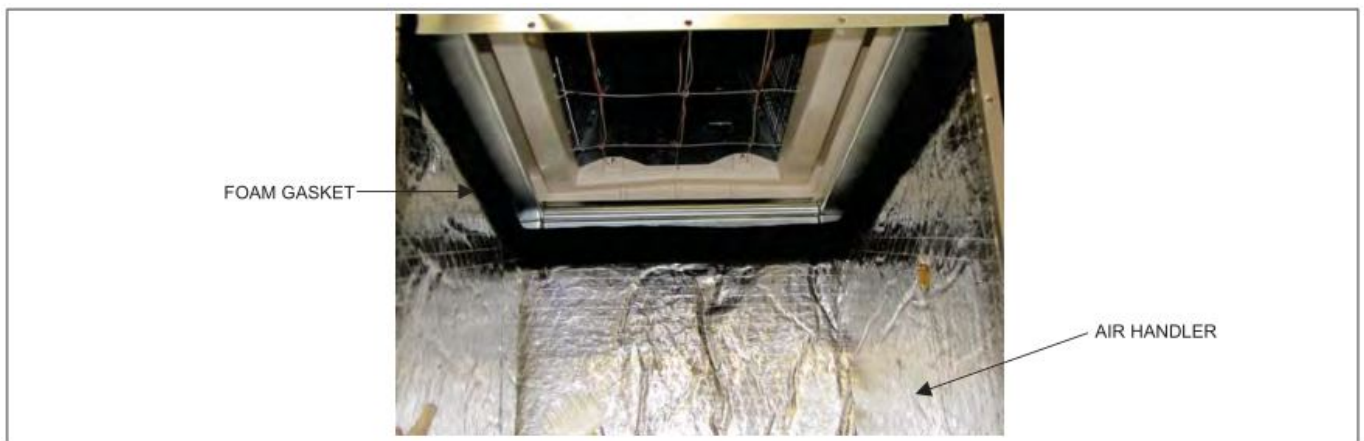
FIGURE 4: Gasket Location
