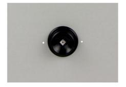
2. Wire the light using the the wiring diagram. Use application specific sealant around the light to prevent any ingress of water. Screw on the bezel.
