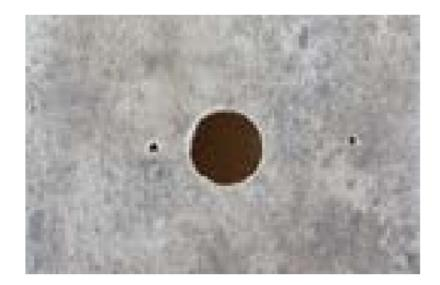
2. Feed the wires through the hole and connect per diagram below. Screw the switch in place.
