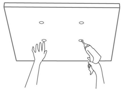
3. • Option A: Knock the plastic anchors into the holes using the rubber hammer. Align the screw holes in the bracket with the holes in the ceiling, and then use the included screws to fix the bracket.
