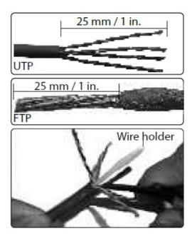
2. Refer to the IDC color codes on the back page to position each wire, and connect it to the patch panel using a Krone or 110D punch-down tool.
