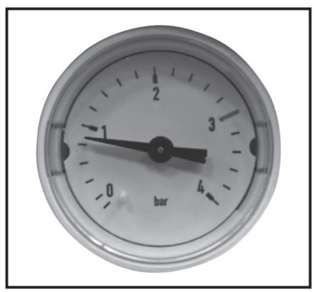
The system pressure gauge indicates the central heating system pressure. If the pressure is seen to fall below the original installation pressure of 1-2 bar over a period of time and continue to fall then a water leak may be indicated. In this event re-pressurise the system as shown below. If unable to do so or if the pressure continues to drop a Gas Safe Registered Engineer or in IE a Registered Gas Installer (RGII) should be consulted.
