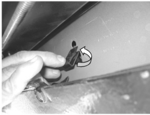
(Fig 5) The Clip Nut Installation
