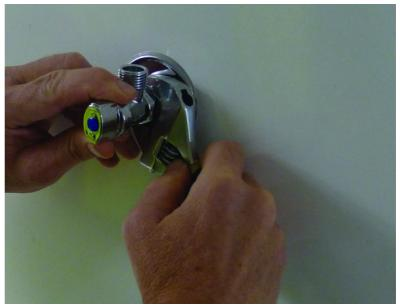
Align stop outlet to the correct position
