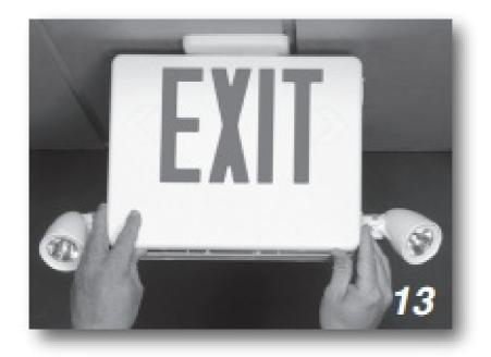
Press the faceplate onto the housing. To install the second faceplate (if required) remove the backplate by pressing in the snaps at the top or bottom of the housing. Then release the two large snaps located inside the housing. Install faceplate.
