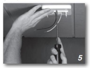
Feed wires through the canopy and fasten the canopy to the mounting plate.
