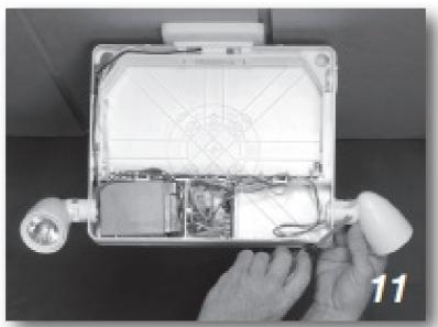
Loosen lamp head adjustment screws. Position lamp heads as required. Retighten.
