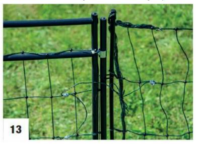
• Connecting the underground cable to the nets on the left and right of the gate
