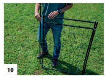
• Place the end/beginning post of the net against the gate and connect the posts
