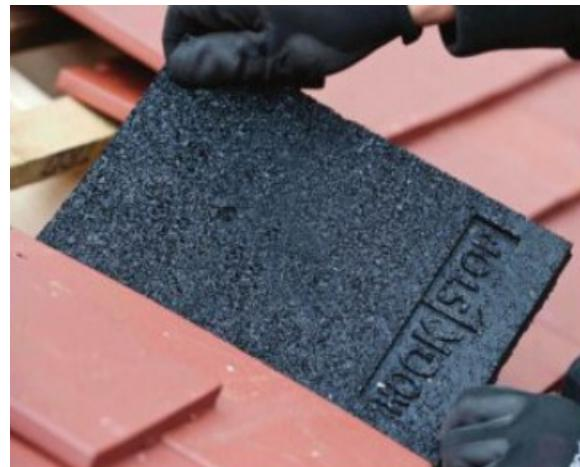
2. Nail the HookStop to the roof batten using two appropriate roofing nails.
