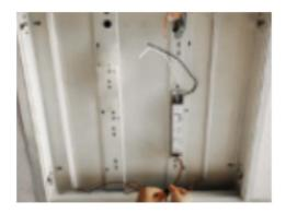
5. Connect driver's input line: Dim +, Dim- and module lines.
