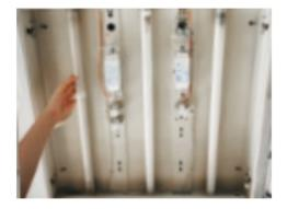
2. Disconnect wires and remove the original fluorescent tube(s) and ballast from the existing fixture. (Recycle tubes according to state specific recycling guidelines).
