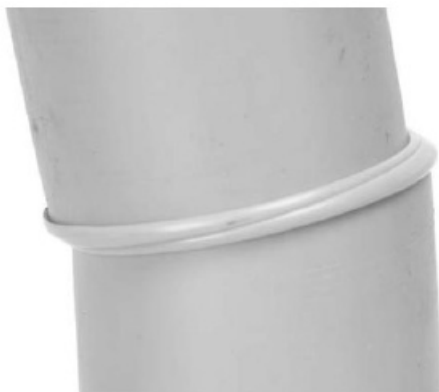
"high-low" pipe alignment. Visually mitered joint.
