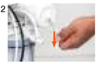
Make sure the incoming feed water is shut off, ensuring the RO filter is depressurized. Disconnect the 1/4" white tubing that feeds the membrane input from the carbon filter.
