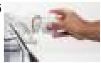
5. Replace the end cap and tighten by hand. If the O-rings are dry, lubricate them with food grade silicone lubricant. Allow system to run for ½ hour before using RO water.
