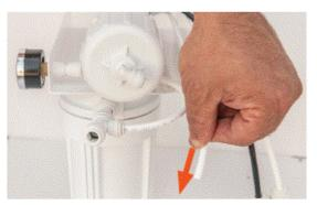
2. Unscrew the membrane housing end cap. Caps can be difficult to remove. Be sure to have a firm grip on the opposite side of the housing. Do not lose the O-ring on the inside of the cap. Each cap has two O-rings.
