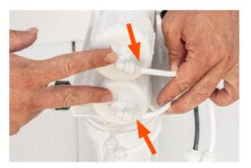
4. Tighten the filter housings by hand, do not use the filter wrench. Do not over-tighten.
