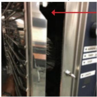
5. With the cleaning brush, push and pull through the entire lengthy of the overflow drain several times. The brush should be inserted at least ten inches (10") into the overflow drain to pass through the entire length of the drain piping. Repeat as necessary until the overflow drain is clean. Ensure that the overflow drain works properly by squirting water into the overflow drain and confirming that the water is flowing freely into the drain receptacle
