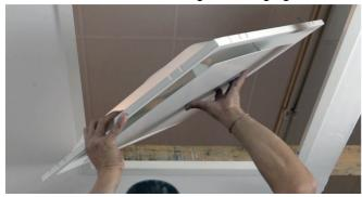
**C.** Once the diffuser is above the ceiling opening, lay the product into the plaster frame or T-Bar grid – **see Figure 2**.
