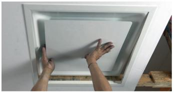
**D.** Attach ductwork to the neck of the diffuser if using flexible duct. This can be done from an adjacent ceiling grid if T-Bar application is used – **see Figure 3**
