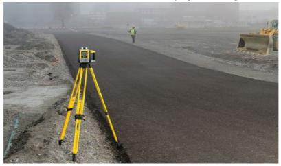
Grade the base course for a road, level its slope, and correct and remove irregularities with the help of GeoMax rotating lasers. They guarantee you repeatable and accurate results in long distances even in the toughest working conditions.
