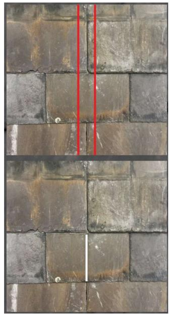
2. You are now ready to mark the top slate, in preparation for cutting.  $Measure\ upwards\ 190mm\ /\ 7.5"\ from\ the\ bottom\ of\ the\ slate\ and\ mark\ with\ a\ line.$
