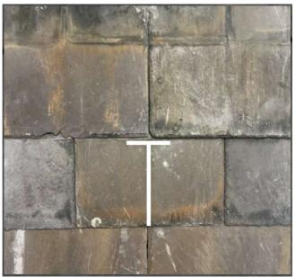
3. To conclude the line drawings for cutting purposes, measure 37.5mm / 1.48" left and right from the centre of the rafter line. Draw vertical lines from the 190mm / 7.5" horizontal line, down to the bottom of the slate.
