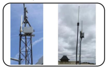
11. Photos show examples of rooftop installation structures for mounting the Gateway. It is the installer's responsibility to select a location where the gateway antenna will be above other obstructions on the roof and will have direct line-of-sight to multiple fixtures that will have LightGrid Controllers on them.
