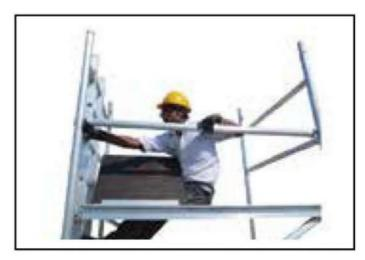
• Step 17 Fit the toe board. Slide the side board into the correct slot in the board. Ensuring the object shouldn't fall and trap door opens fully.
