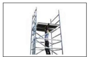
• Step 16 Sitting through trapdoor fit two horizontals on both open sides of the platforms.
