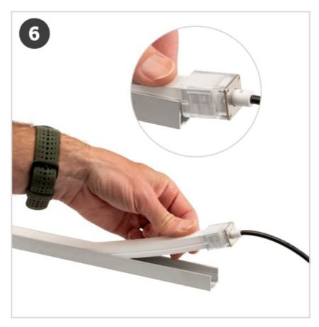
7. Press the strip light into the installed SRP-MNT Hardscape Mount. The ideal placement is one mount every 20" (508 mm) or less.
