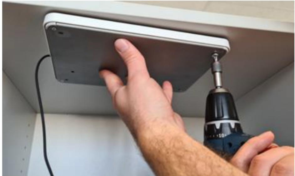
Figure 10: Under table mounting
