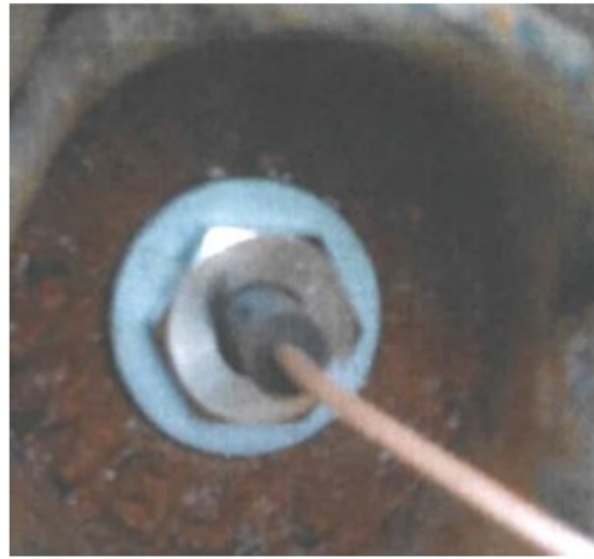
Figure 21. Thread antenna into position and secure in place with supplied nut and a suitable washer
