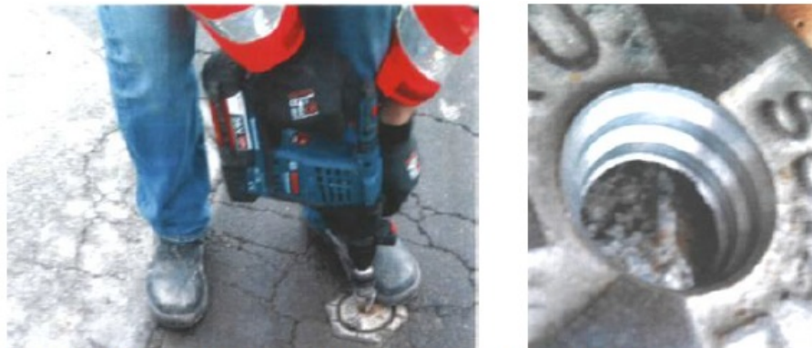
Figure 20. Drill hole and recess in chamber lid
