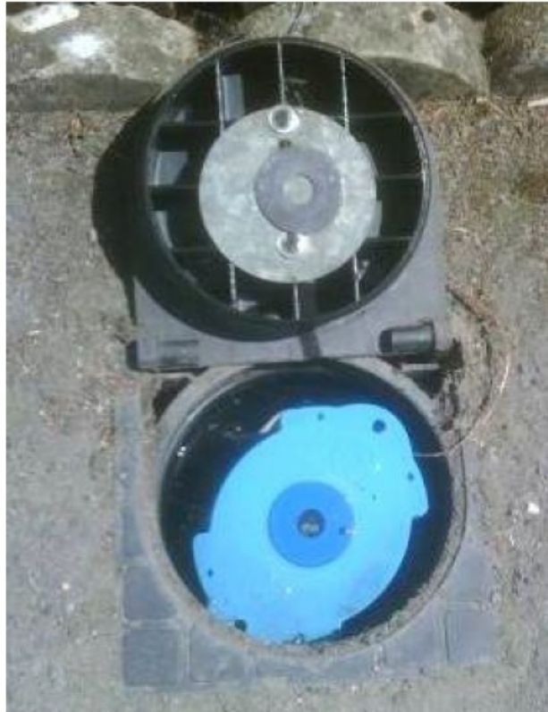
Figure 16. Logger mount using a plastic tube example
