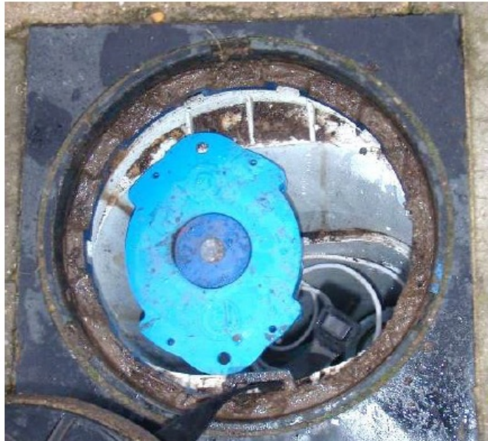
Figure 14. Logger in Talbot round lid box example
