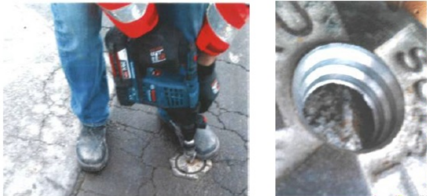
Figure 30. Drill hole and recess in chamber lid
