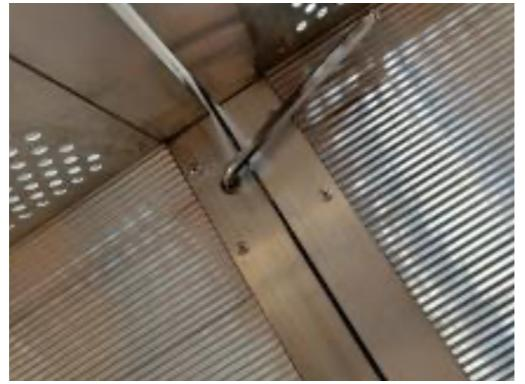
5. Using an Allen key, turn the wall latch anti-clockwise until it has grabbed onto the adjacent unit and can move no further.
