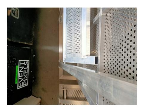
Using an Allen key, turn the latches clockwise to undo, making sure to turn all the way to release each part from the other. Always start from the outer-most units first. Loosen nut of the floor holding screw, and remove the screw. Lift the smaller frame behind the wall and carefully push forward on the wall part from near the base, while standing on the floor and lowering the wall towards the collapsed position, making sure the smaller frame folds in with it
