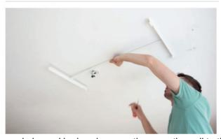
2. After you have drilled the holes and plugged in dowels screw the mounting rail to the ceiling.
