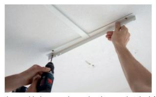
3. Hang the LAVA® one-sided in the provided suspension and make sure that the LAVA® is correctly locked in
