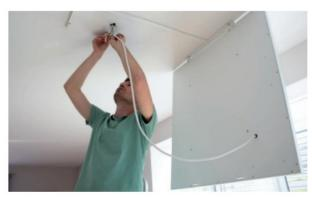
5. Hold the LAVA® firmly in the suspension and push the other side of the device up to the mounting rail.
