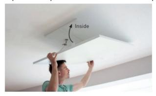
6. Press the LAVA® slightly upwards and insert the two secu-ring pins to fix the device in the mounting rail.
