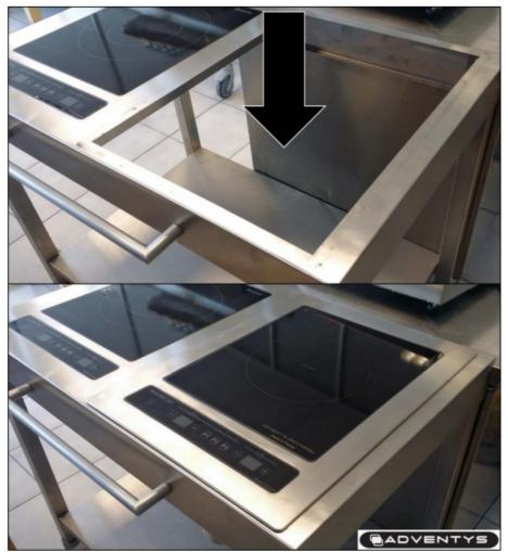
Carefully place the unit into the opening to check fit. If any adjustments to the opening size are necessary, make them before proceeding to the next step.
