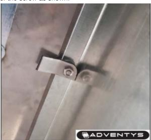
Thread the nut over the screw and hand tighten. Do this for all four locations, and then tighten firmly being careful not to over tighten.
