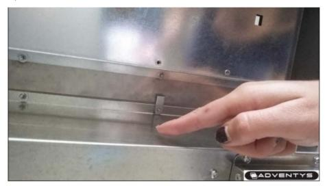
Place the mounting bracket over the screw as shown.
