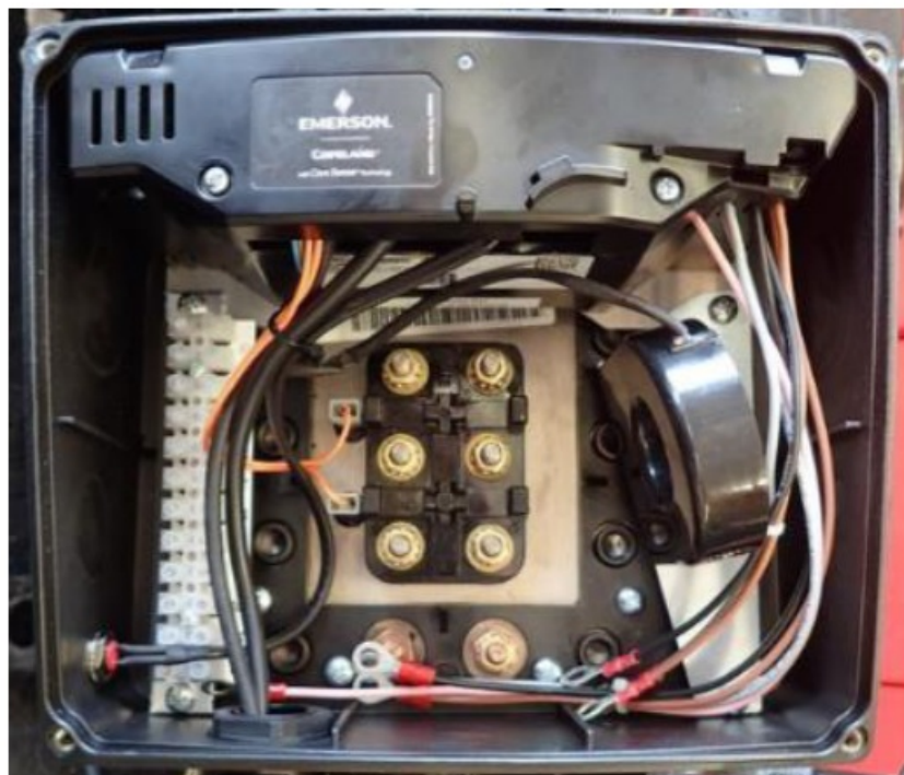
Figure 2: Next Gen CoreSense inside the terminal box
