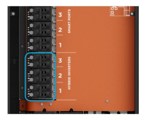
Reference the table below for wire size and torque recommendations when connecting the hybrid port wiring.
