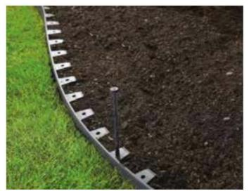
2. Hammer anchoring spikes through tabs to secure the edging. Typical installations require one spike every 10 tabs. Additional spikes are available separately.
