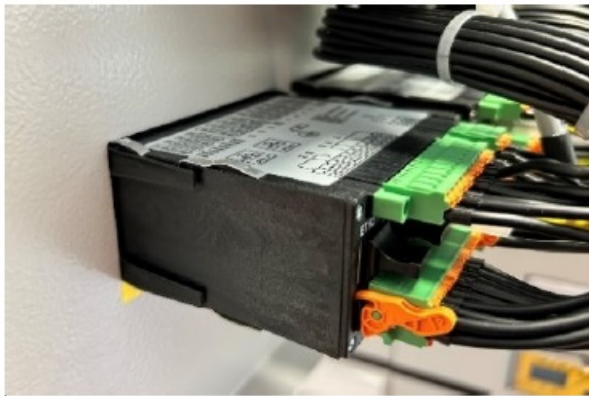
EOR-3DS in control panel cut out
