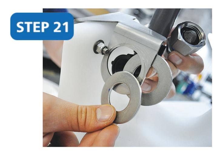
Install the stainless steel adapter parts by placing one washer on the inside of the cart bracket and one on the outside. Thread the stainless steel hose adapter onto the elbow and tighten with a box crescent wrench for a snug fit.
