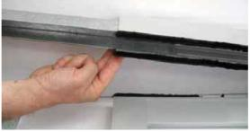
16. If the width of the mobile wing is greater than 1000 mm, insert reinforcement 4173 into profile 3820, as shown in the diagram.
