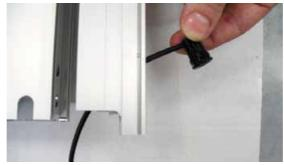
7. Insert the photocell [25], which detects the opening of the mobile wing, into profile 3831, as shown in the diagram.
