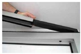
15. Fasten detail [3] to profile 3820, as shown in the diagram.
