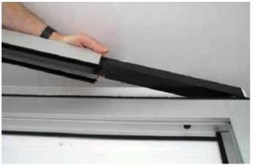
14. Insert profile 3820 into detail [3]. as shown in the diagram.
