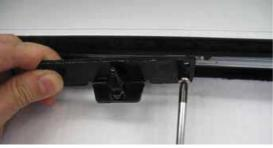
17. Fasten profile 3924 to the hinge side vertical upright, as shown in the diagram.
