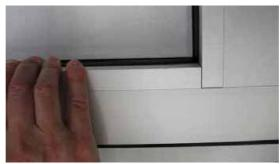
28. With PAM45M profiles, insert the glass-blocking profiles [8] onto the mobile wing until they click, as shown in the diagram.
