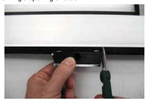
13. Trim the brush SPAZ4811 where it connects with detail [5], as shown in the diagram. Note: Be sure to take note of the wing's opening direction.
