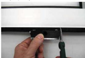
13. Trim the brush SPAZ4811 where it connects with detail [5], as shown in the diagram. Note: Be sure to take note of the wing's opening direction.
