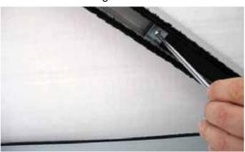
Note: during the installation of the fixture, in order to obtain the proper horizontal position of the mobile panic wing, loosen the fastening screws and adjust the screw shown in detail 3], as shown in the diagram.
