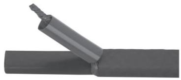
3. Cut and remove the inner insulation 10 mm from the end.
