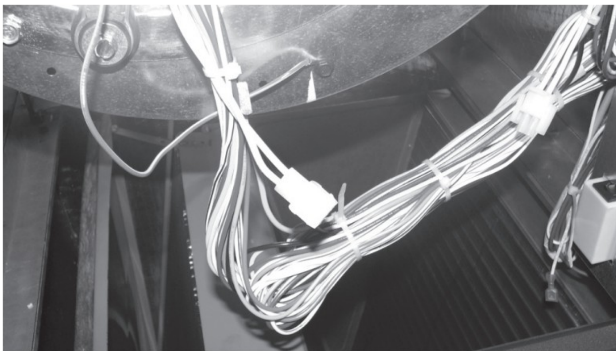
Figure 12: Install Two Pin Jumper Plug
