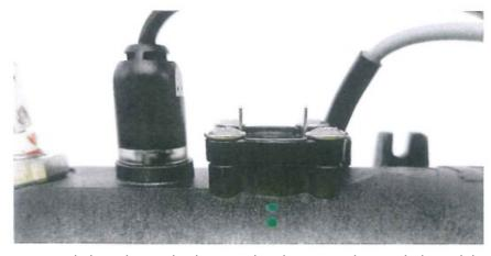
21. Remove the earth screw and place the earth wire onto the element and screw it down tight.
