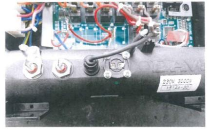
8. Undo the earth screw and remove earth wire. Replace earth screw into tube s to not lose it
