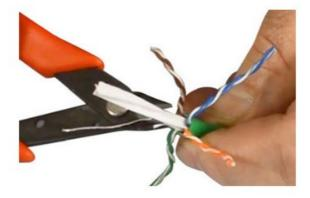
**STEP 4**Trim center spline/pair separator as close to the cable jacket as possible without nicking any of the wire conductors.
