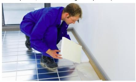
6. **Fig. 6:** Where required cut individual pipe channels using the Speed Up hot wire cutter.
