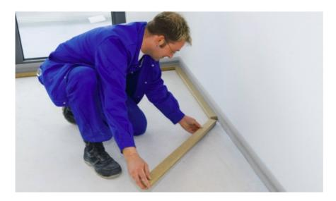
2. **Fig. 2:** Following the layout, begin the installation in one corner with a Speed Up header panel.
