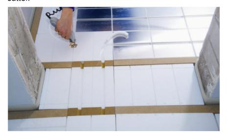
7. **Fig. 7**: Support battens in thresholds should be screwed down.
