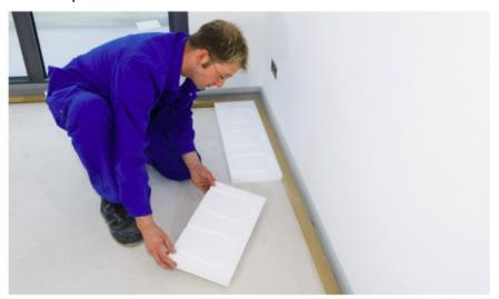
3. **Fig. 3:** Place the Speed Up heat panels (CZ: pipe distance 250 mm, EZ: pipe distance 125 mm). Fill gaps and unheated areas with blank panels.
