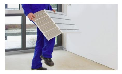
Fig. 5: Light constructions (e.g. laminate/engineered timber or strong board constructions laid directly on the heat panels): rooms > 12 m² glue all perimeter and header panels, rooms < 12 m² glue all panels (recommended).</li>
