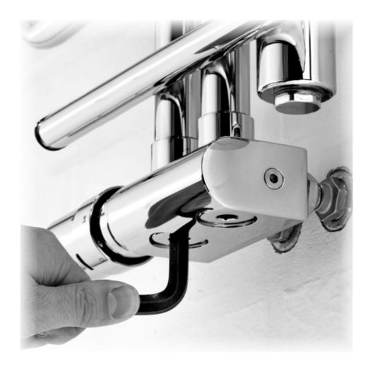
• Tighten valve to radiator.
