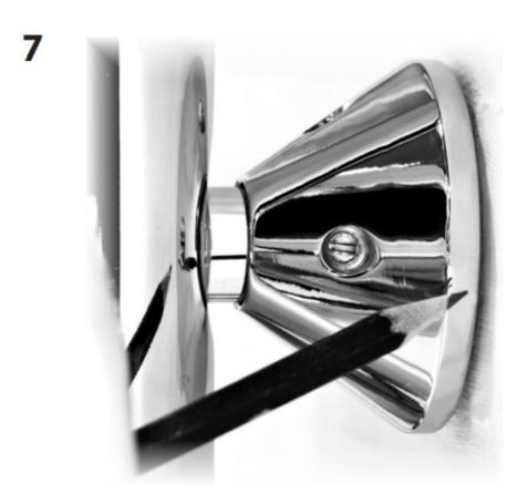
Mark position and mount radiator on wall.
