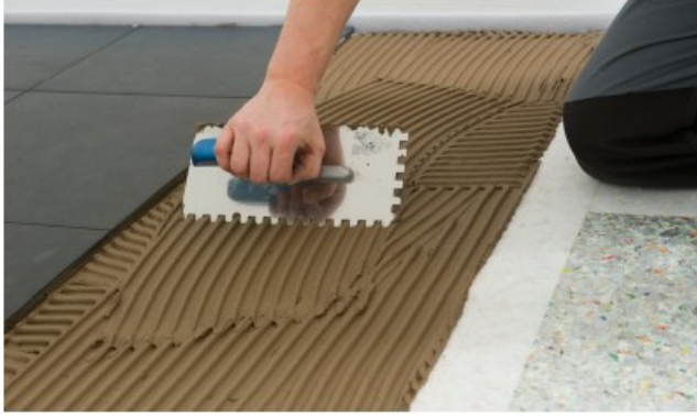
Fig. 3: Number of notches on the tile adhesive comb/trowel depends on the tile size: · 8-notch trowel for tiles from 10×10 cm to 30×30 cm · 10-notch trowel for tiles up to 60 cm x 40 cm
