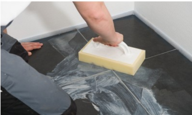
Fig. 9: Having applied the grout use a sponge board to clean the tiles diagonally to the grout direction.
