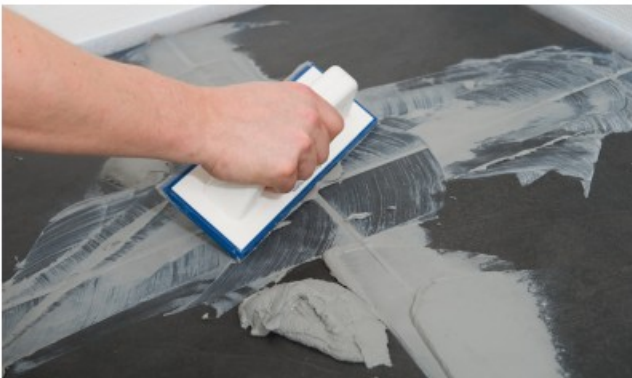
Fig. 8: Grout the area after 24 hours with Mapei ULTRA COLOR plus.
