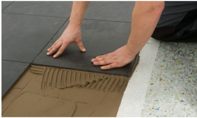
Fig. 6: Press tiles down firmly eliminating any air trapped in the process. Ensure that the depth of the bed is at least 4 mm.
