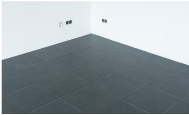
Fig. 10: It is safe to walk on the tiles after 24 hours. The floor heating can be turned on 7 days after grouting at the earliest.
