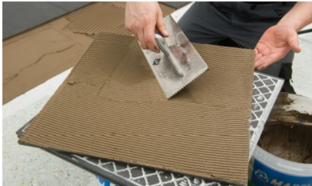
Fig. 4: Also fully apply tile adhesive to the back of the tile.
