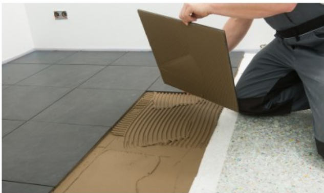
Fig. 5: Using the buttering- floating technique press the tiles on to the prepared floor.
